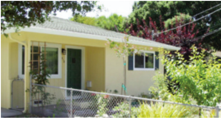
Before and after of Casanova house.
